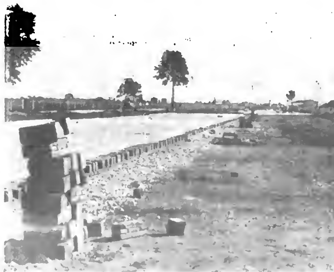
First Sample of Brick Surface Laid at Motor Speedway
